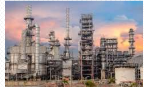
Heavy & Complex Structures
