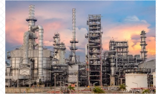
Heavy & Complex Structures
